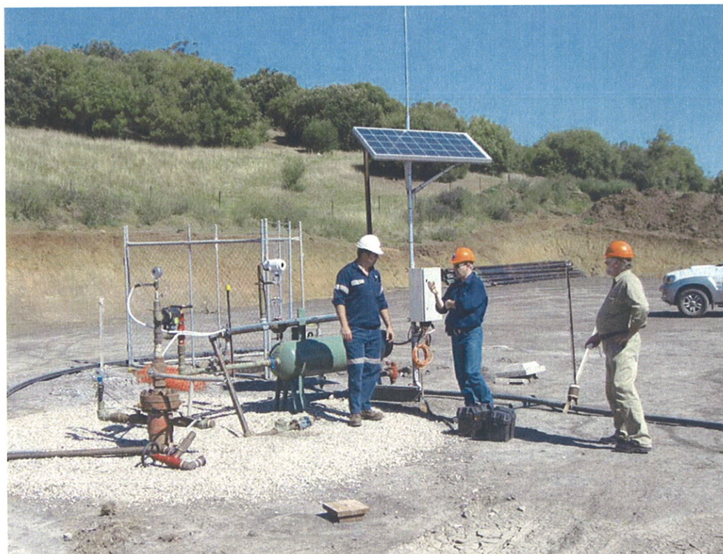
Figure 8: Gas wellhead in operation
